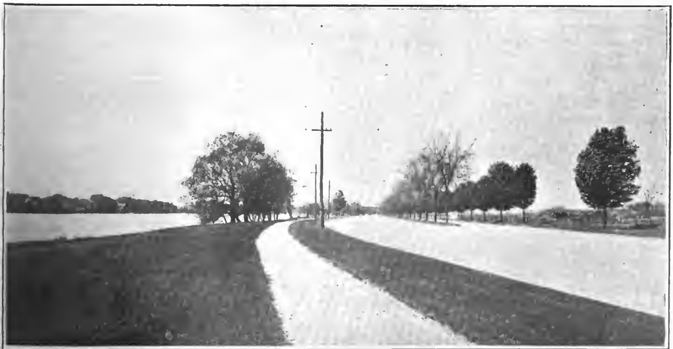
Example of a Fine Road Surface, as Prepared for Massachusetts, Showing Separate Road for Heavy Traffic
